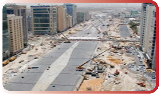
Samsung C&t Deep Tunnel Project-uae
