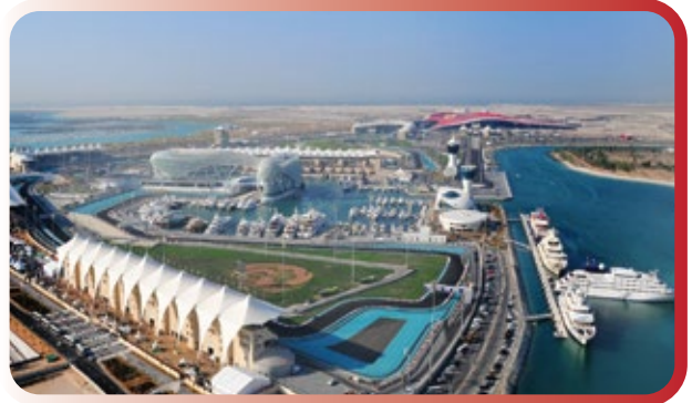
Control & Application Yas-marina Cercit Project-uae
