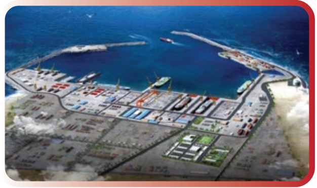
Daewoo Ship Repair Yard-oman
