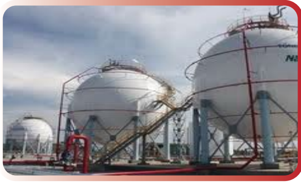
Daewoo Gas-tank Project-nigeria
